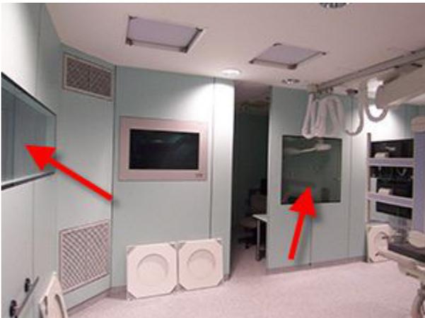
*EMI/RFI shielded mesh foil window example*
