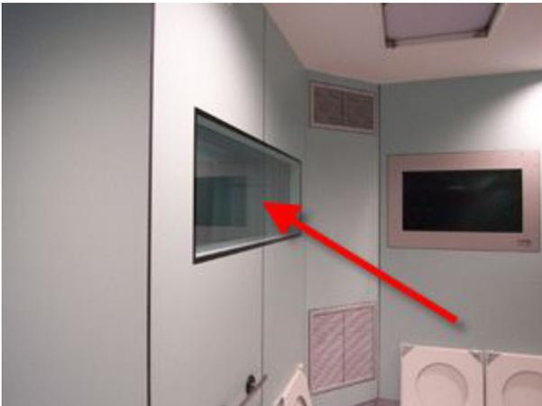
*EMI/RFI shielded mesh foil window example*
